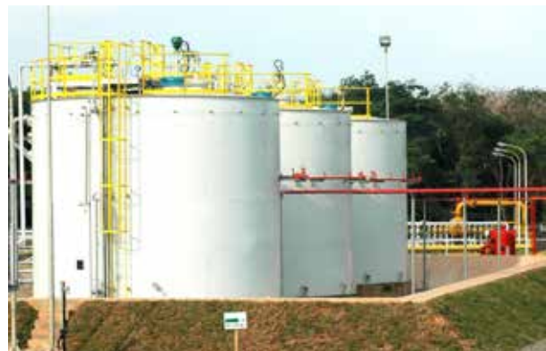
Concrete berms can contain catastrophic tank failures.
