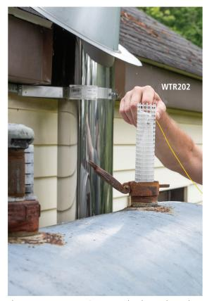
The PIG Water Hog contains a superabsorbent polymer that will absorb 200 times its weight in water from the bottom of your fuel tank, providing you with uncontaminated fuel for work and recreation.
