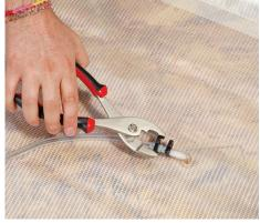
4. Slide clamps over the barbed fitting and pinch together with pliers to secure the clamp onto the hose and fitting.
