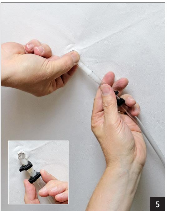
Connect drainage hose to drain elbow using barbed coupling. Apply clamps to both connections.
