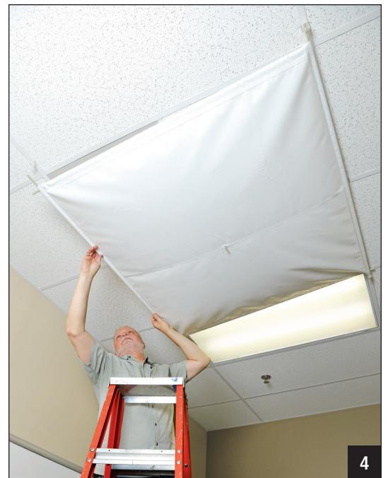
Hang opposite rod in remaining grid clips. Make sure the shorter rods are resting on top of the longer rods.
