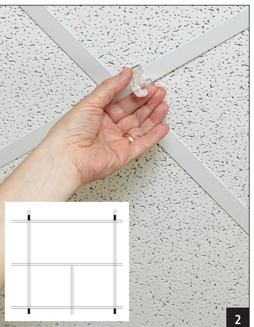
Install four clips onto ceiling grid at corners of 4' x 4' layout (Diverter will cover four 2' x 2' tiles or two 2' x 4' tiles)
