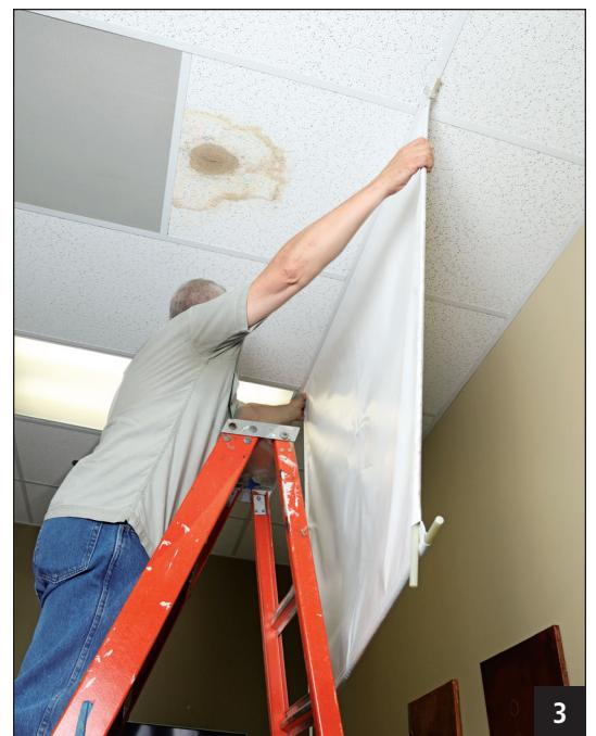
Hang one end of the diverter by snapping a long rod into two grid clips. (Position tarp so drain will face downward after completion of next step.)
