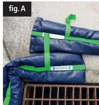
When using multiple units, the socks should be run continuously, without gaps. The easiest way to accomplish this is to overlap the socks (fig. A) or stack them on top of each other (fig. B).
