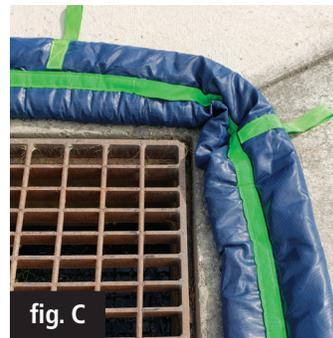
90° bends can be accomplished by creating a crease in the inner chamber (fig. C & D)
