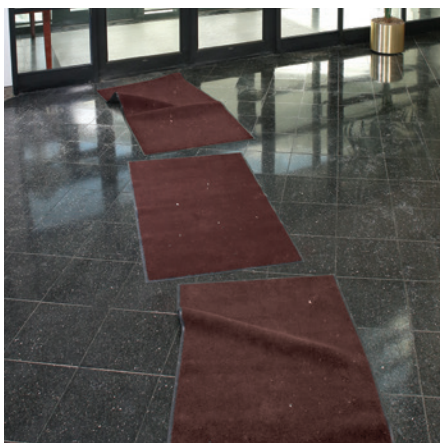
Multiple mats shift out of position producing gaps and wrinkles that cause slips and trips.
