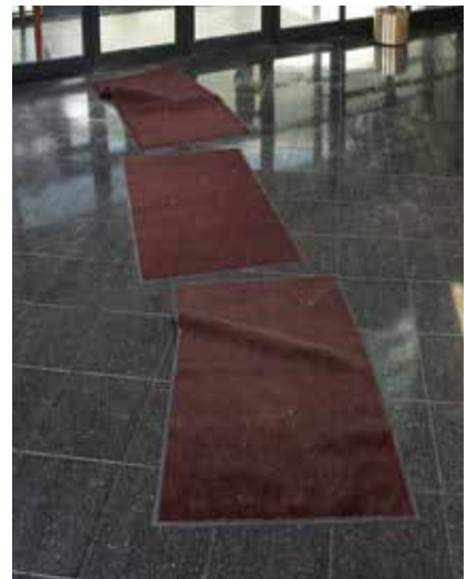
Carpeted floor mats shift because they depend on weight to stay put.
