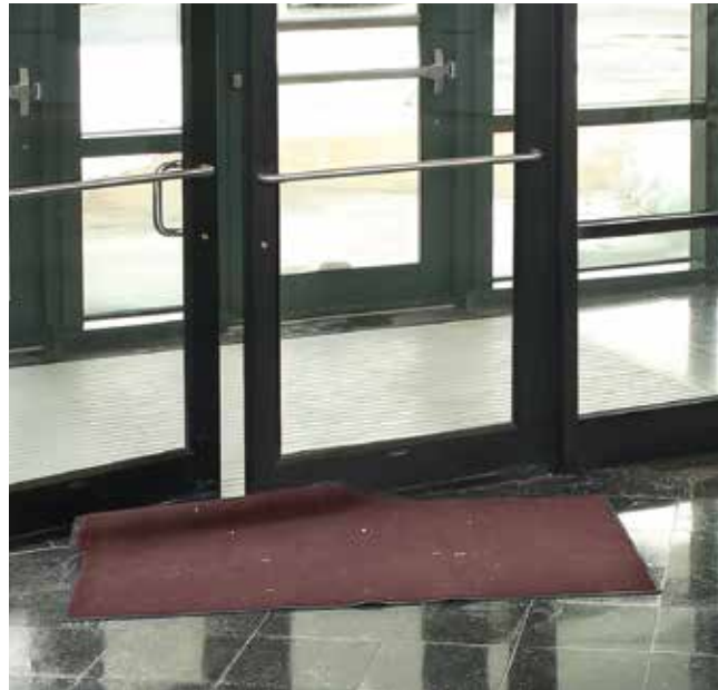
Bacon mats detract from a facility's appearance.
