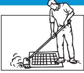
1. Sweep the area surrounding the drain and remove debris to ensure a proper seal.
